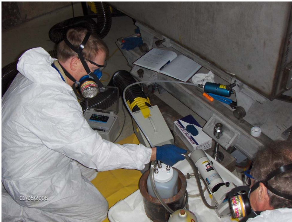
Figure 1. Mercury draining operations
